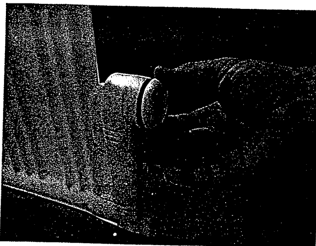
2 Drag loss termostatratten
